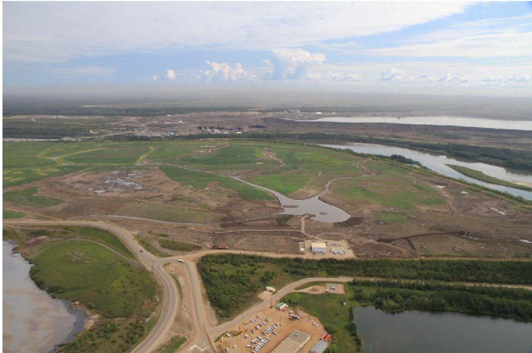
Figure 3: Suncor Energy's Wapisiw Lookout (formerly Pond 1) in August 2010. In time, Suncor expects this land will become a productive mixed wood forest and wetland environment. Over the next two decades, Suncor will closely monitor progress on the site, including the growth of the 630,000 shrubs and trees planted in 2010.
